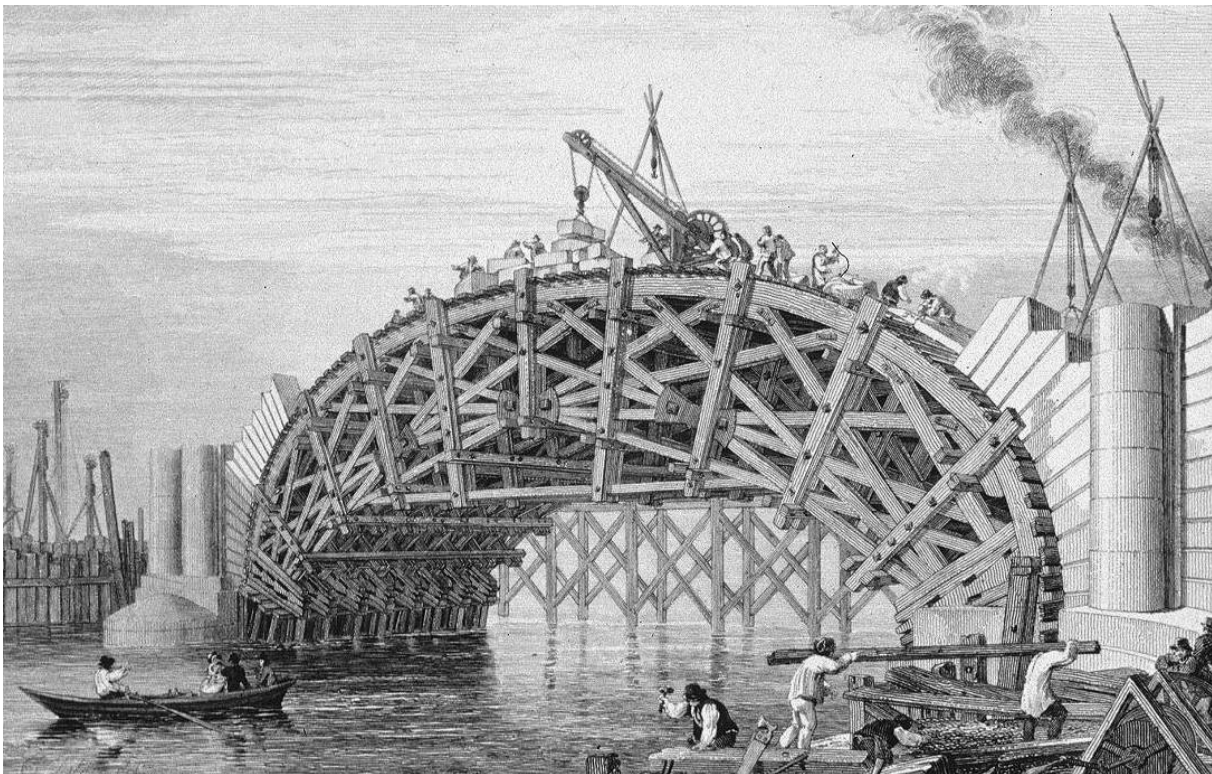
Figure 4. Wooden Centring used in the Construction of the Waterloo Bridge
