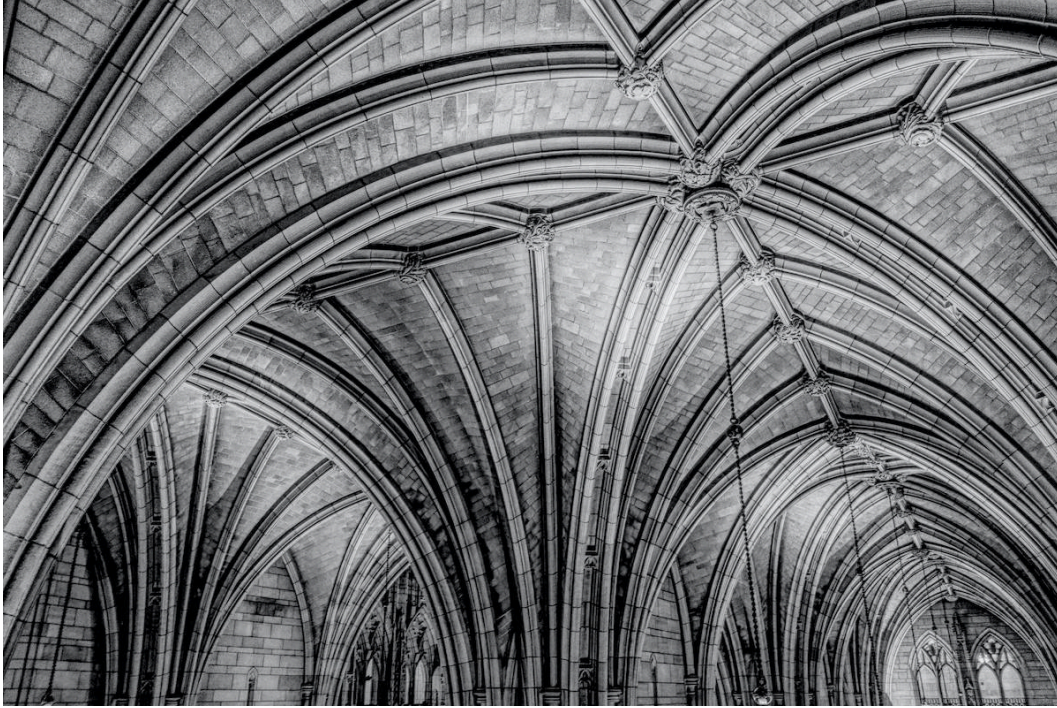
Figure 3. A Vaulted Ceiling 3
